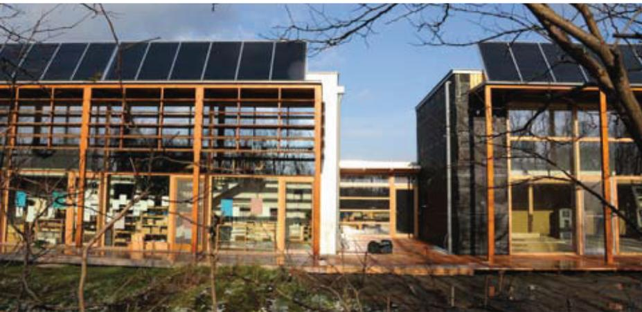
This is module 2 of the Montessori Campus in Marchegg, Lower Austria, which was planned by the architect Martin Rührnschopf from Vienna. The module is designed as an active solar house with a solar fraction of 85 %. Rührnschopf wants to compare it with module 1, which is built as a passive house and heated using a heat pump.
